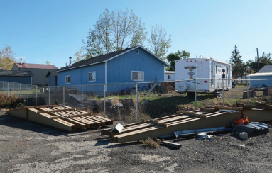
APPROX. 17'X31'X80' DISMANTLED HANGER BUILDING
