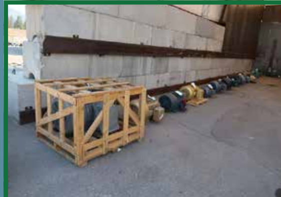
LARGE QUANTITY OF SPARE DRIVES & SPARE MOTORS
