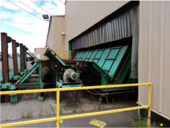
Incline lumber transfer
