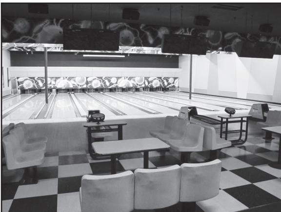
(23) Bowling lanes w/synthetic tops, approaches, pin decks, AMF 82-70 auto pin setters, gutters & bumpers, masking panels, BRUNSWICK 2000 ball returns, QUBICA/AMF score keeping touch pads, scoring monitors, pin setter parts and equipment
