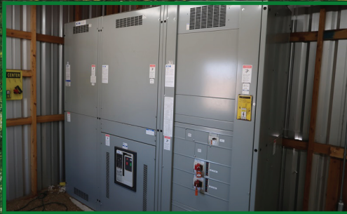
2014 CH EATON 2,000 AMP 3-SECTION POW-R-LINE SWITCHBOARD
