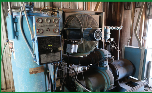
2002 QNW 1011-D ROTARY SCREW COMPRESSOR
