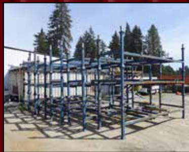
SHOP BUILT RACKS
